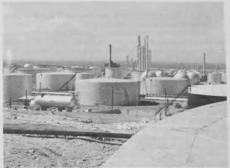
Tanks of varying shapes and sizes can be seen from top of a cone roof tank.
